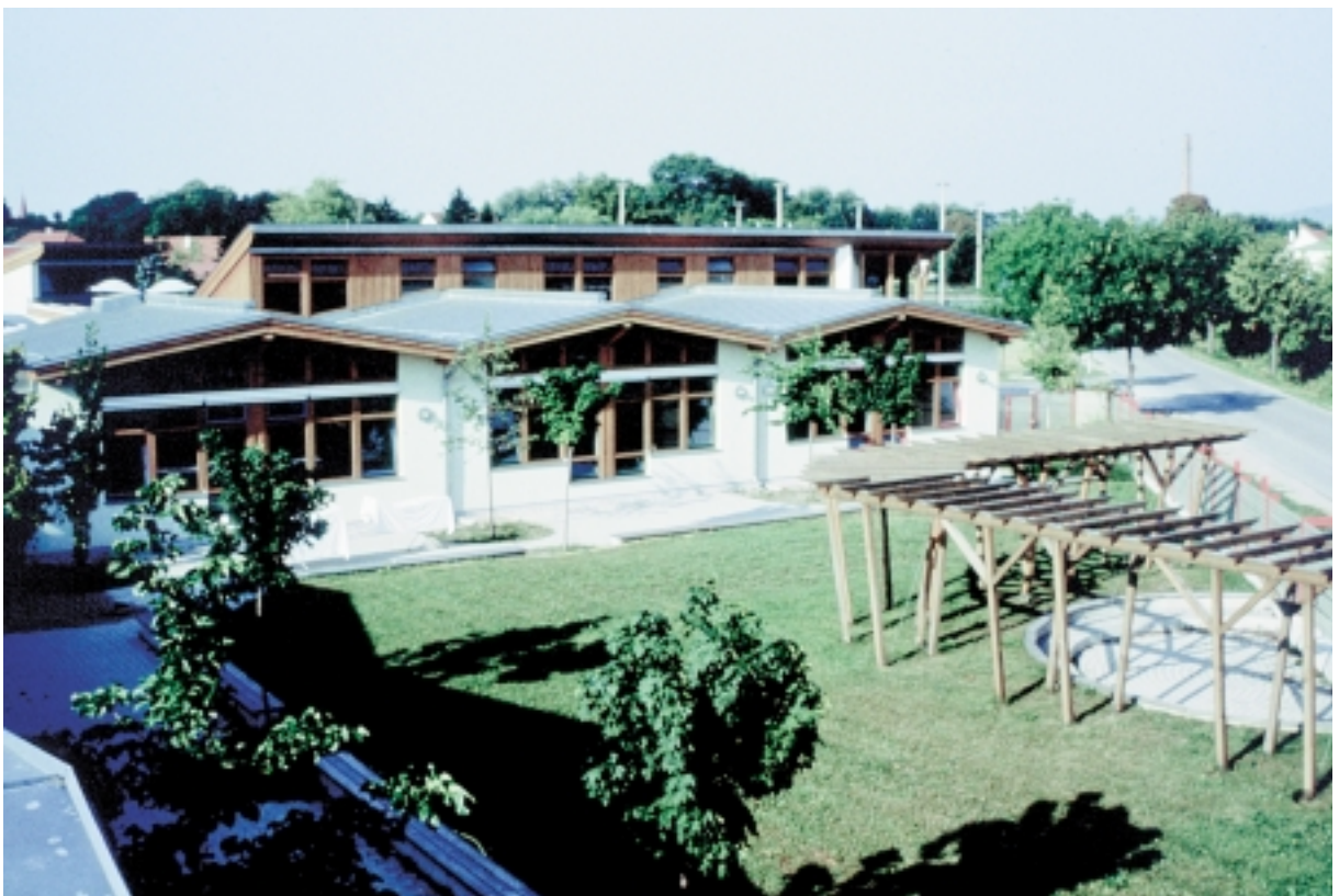
Picture 2 - South oriented classroom windows facing the recreation yard.
