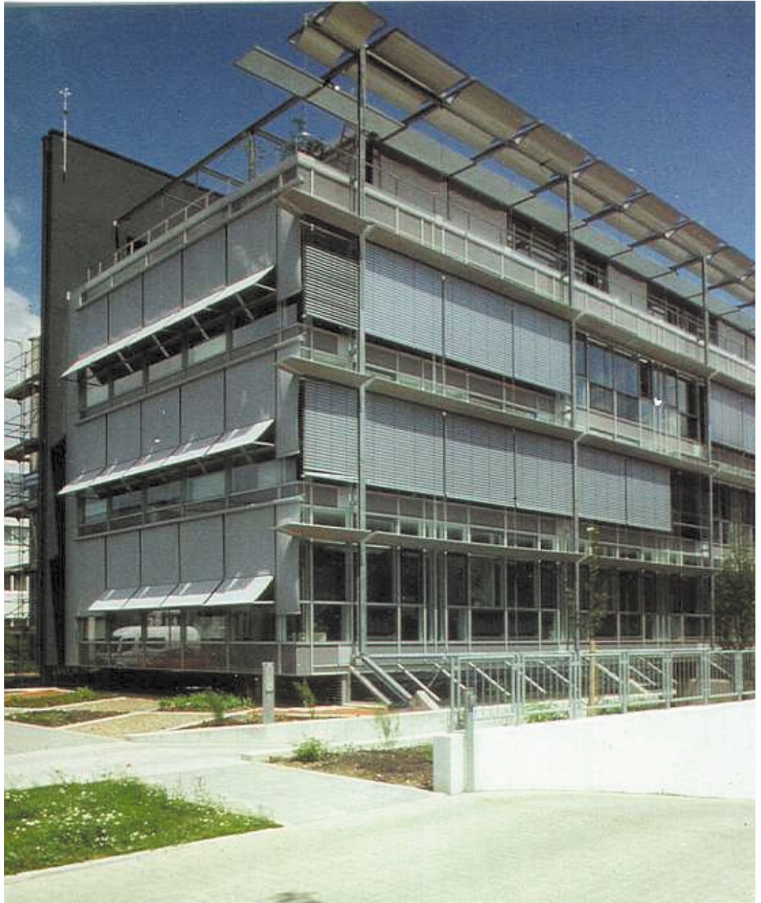
Picture1 - South west elevation of the facade. South facade with light shelves and air collectors.
